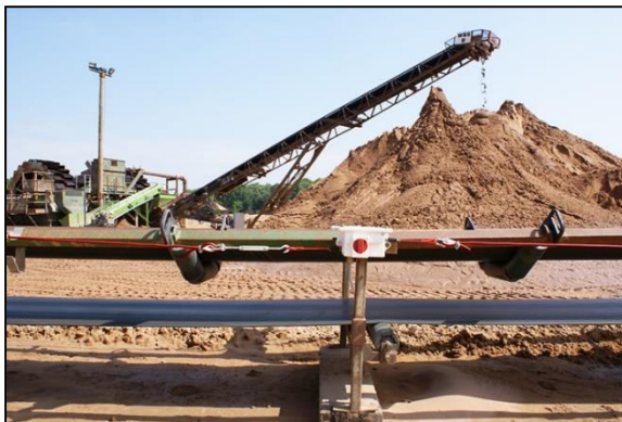
Open Conveyor Installation at Sand and Gravel Facility
